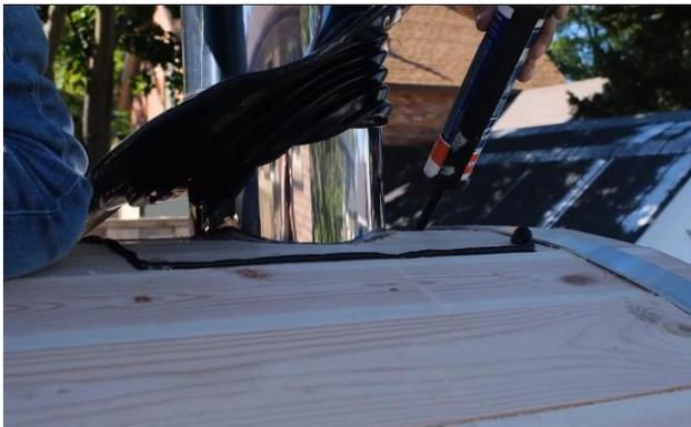
Lift the boot out of the way and apply the included roof sealer on the inside of the outline.
