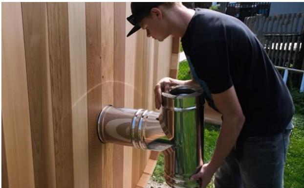
Insert the "T" chimney piece through hole in back of sauna and through the rear wall heat shield on the inside of sauna and into the back of stove.
