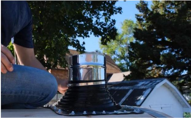
Place the hose clamp over the boot and tighten the screw.
