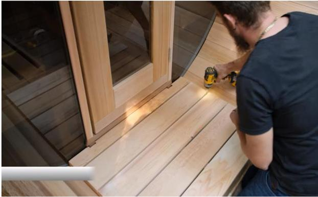
Place the porch floor with the notches for the door facing the door/
