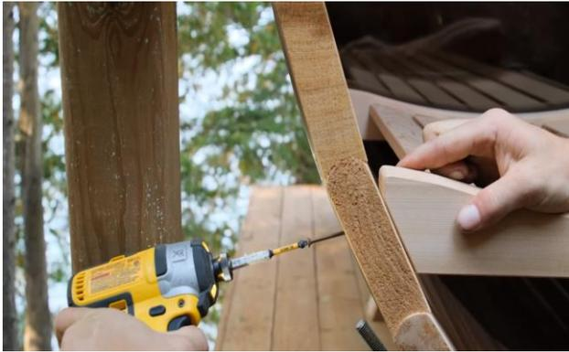
Use a 2 ½" (64mm) screw to fasten the front and the back of the porch seat screwing through the side stave into the seat supports.
