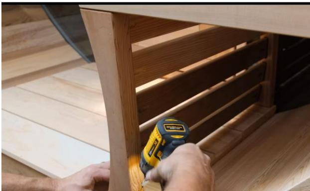
Secure to the floor and wall under the seat using 2 ½" (64mm) screws.
