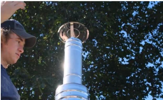
Insert the short chimney piece into the thick chimney piece, followed by the cap piece.
