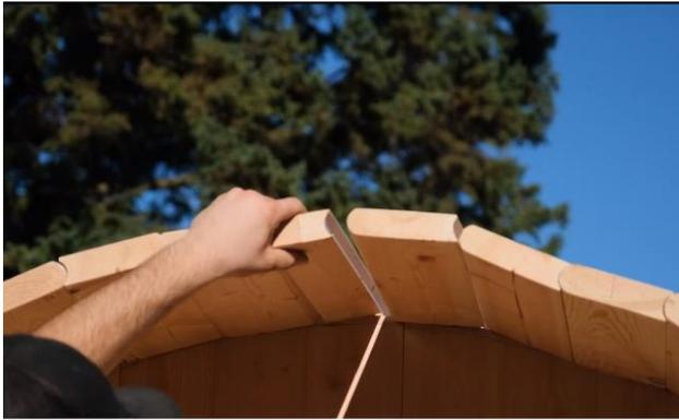
In your sauna package you will find a spacer stave that is square on both sides that is only required if there happens to be a “gap” after installing all the staves like in the picture on the left.
