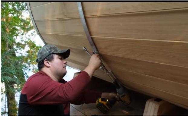
Feed another band over and under the sauna and secure it with a rod and nut.
