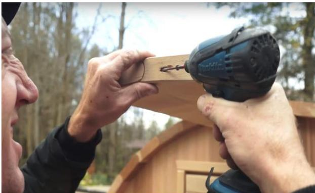
Fasten each cove piece to the next through the pre drilled holes on the front of each piece using a 2 ½" (64mm) screw.
