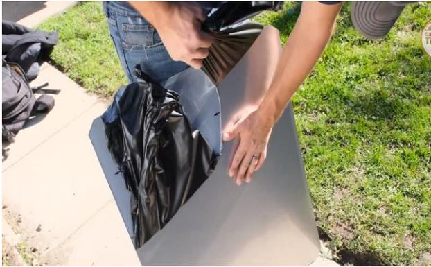
Remove all protective film from stainless steel parts and the plastic wrap from stove pipe pieces before installation.
