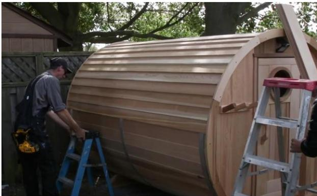
When you have installed the bevel siding up to the top, start installing the other side following the same process.
