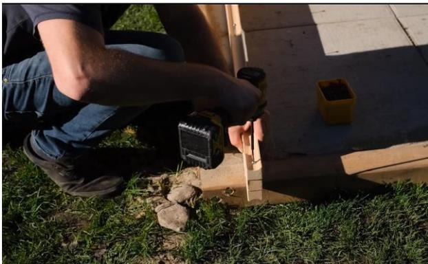
Now screw the other side of the top stave back to the other half top stave and it should now make a “V” shape when wedged with the last stave on the sauna.
