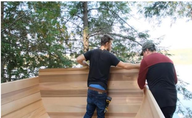
Place the window support piece onto the back wall.
