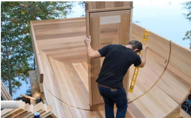
Place the door panel into the front groove of the sauna and ensure it is level.
