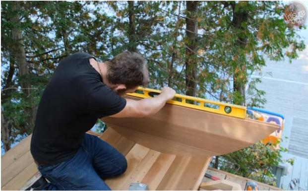
Place the back bottom wall panel centered into the groove at the rear of the sauna and ensure it is level.
