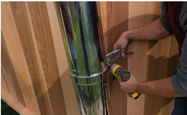
Attach a support strap around the connection and tighten up.
