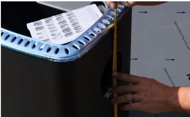
Measure the height to the middle of the opening on the back of stove. (22") (56mm)
