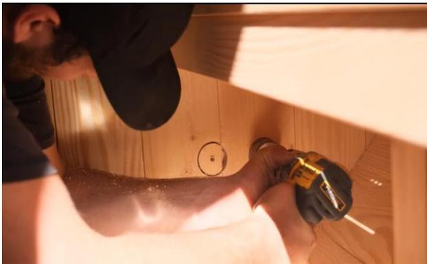
Drill out with a 2" (51mm) hole saw.
