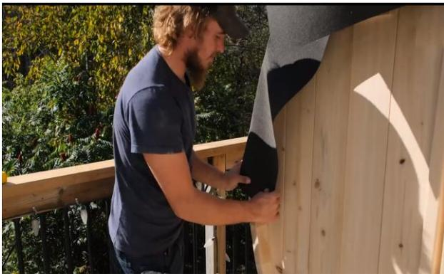
Fold the ice & water shield over the front of the staves.
