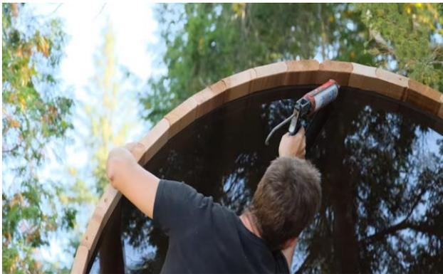
Use the caulking to seal the seams on the outside of the rear window.
