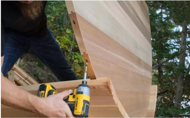
Place the middle back wall panel onto the bottom panel and secure with 2 ½" (64mm) screws in the pre drilled holes.
