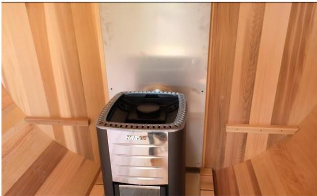
Ensure the rear wall heat shield is level and secure with 6 - 1 ½" (38mm) screws through the drilled holes.
