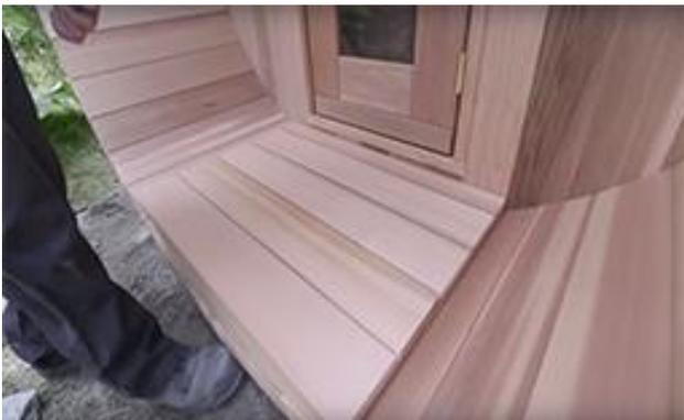
If the porch option is selected, start by installing the floor ensuring it is level.
