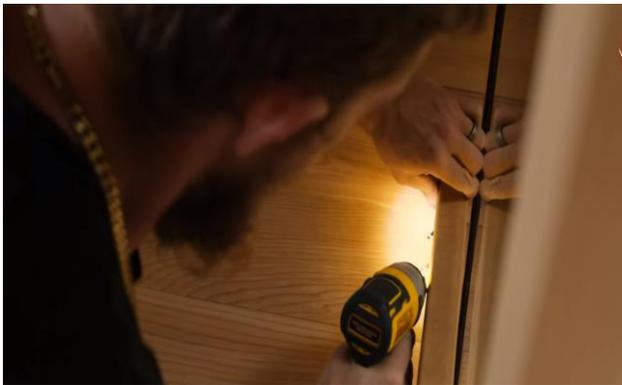
Repeat the process with the large support at the front of the sauna and secure to the wall of the sauna with 2 - 1 ½" (38mm) screws.
