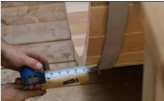
Again, ensure the front band is 2" (51mm) from the edge of the sauna all the way around.
