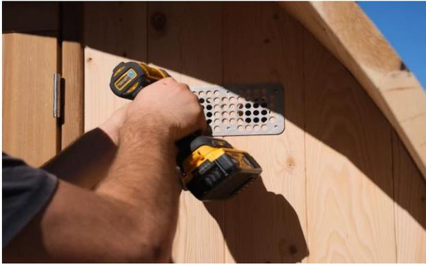
High on the front wall, repeat this process and mount the vent cover on the outside of the sauna.
