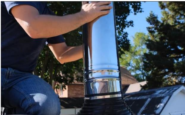
Place the 2<sup>nd</sup> insulated chimney piece over the first.
