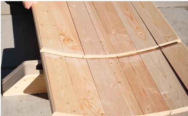
Place 3 staves on either side of the bottom stave and align the grooves.
