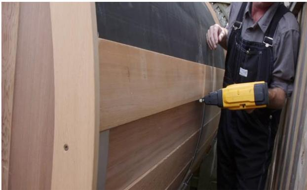
Fasten the bevel siding to the sauna using a staple gun with 1 ¼" (32mm) crown staples.
