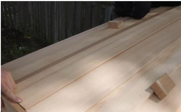
Use one last piece of the bevel siding to overlap the 2 sides.
