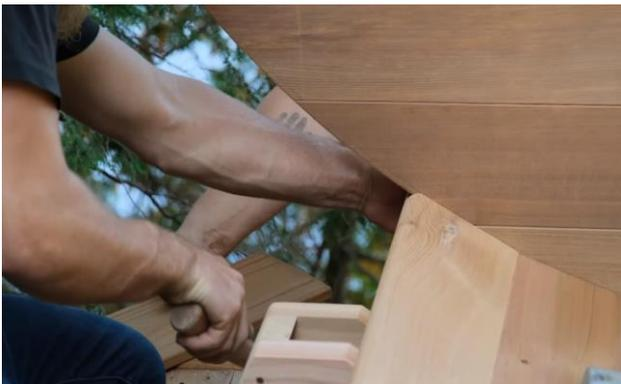
Secure every 2<sup>nd</sup> stave on the bottom of the sauna with the provided nails to hold staves in place.
