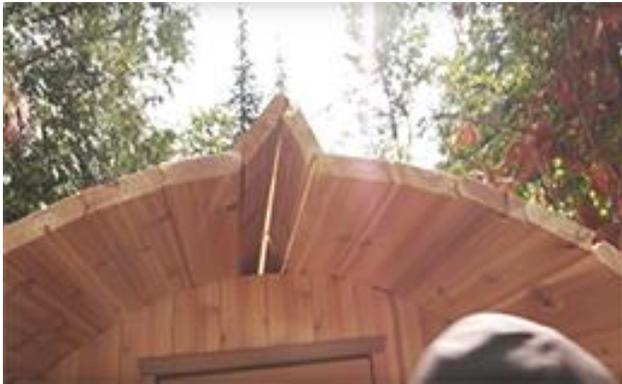
If the staves do not close together in a uniform shape, you will need to add a n include spacer
