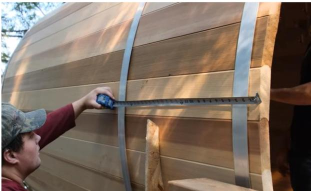
Place this band directly over the front wall panel making sure it is even all the way around the sauna.
