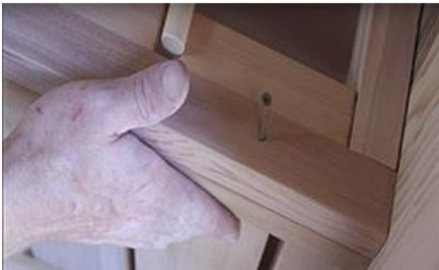
Ensure bench is flush with the bench support and secure with 2 ½" (64mm) screws in the pre drilled holes.
