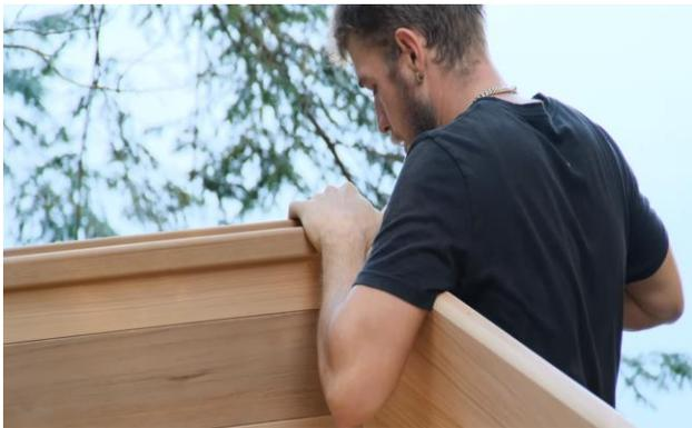
Place another stave on each side of the sauna and secure into the wall using 2 ½" (64mm) screws.
