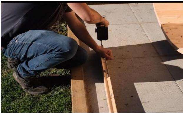
To make the top stave narrower, start by removing all of the screws from the top stave.
