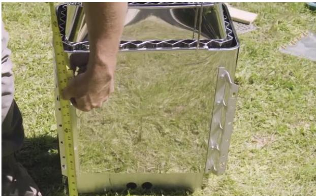
Measure the height of the mounting holes and add 6".
