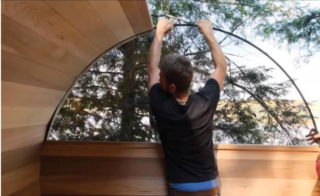
Slide the rear half moon window into the groove on the back wall and make sure it is snug into the wall.
