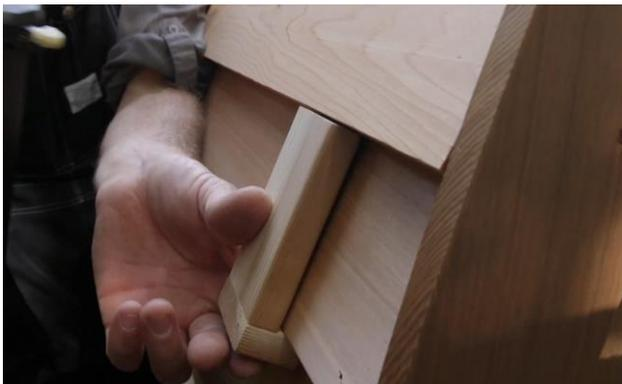
Use the provided spacing blocks as shown to get the correct placement of the next piece of bevel siding.
