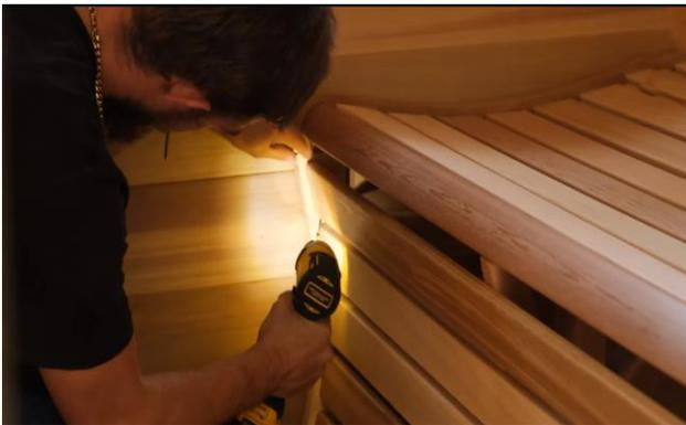
Secure the front enclosure the wall and the bench supports using 1 ½" (38mm) screws.
