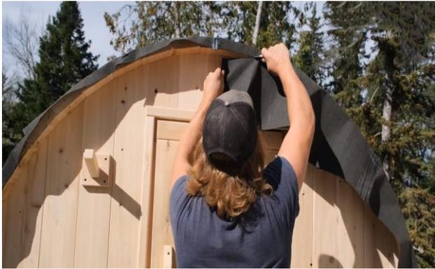
Using a utility knife, cut off the excess rubber flush to the edge of the staves on the front and back of the sauna.
