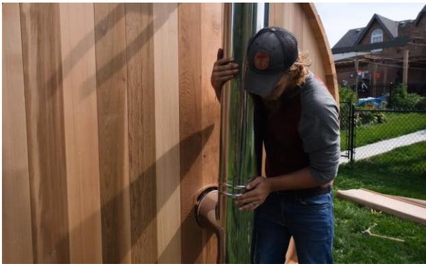
Attached assemble chimney pieces to the "T" coming out the back of the sauna.
