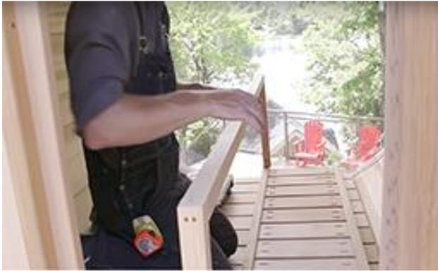
Using the pre drilled holes, assemble the lounge bench support to the longer front lower bench wall using 2" (51mm) screws.
