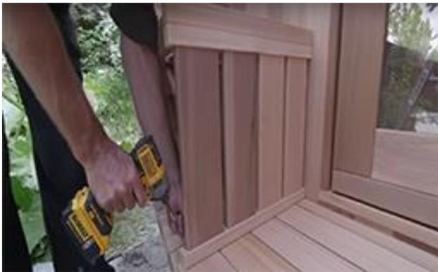
Fasten bench to floor and sauna wall using 3 - 2 ½" (64mm) screws on the top and bottom.
