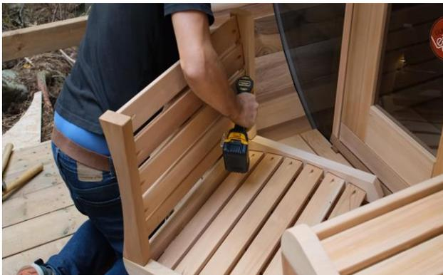
Flip the porch seat upside down and secure the front porch enclosure to the seat ensuring the contour is facing the right way using 2 ½" (64mm) screws in the pre drilled holes.
