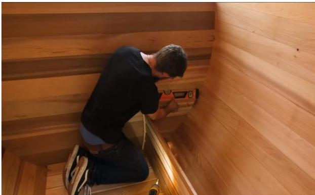
Place the small support bracket onto the rear wall of the sauna and ensure it is level.
