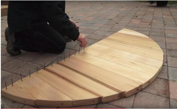
Line up the cove pieces starting with the smallest pieces on the end and working towards the middle forming a semi circle.
