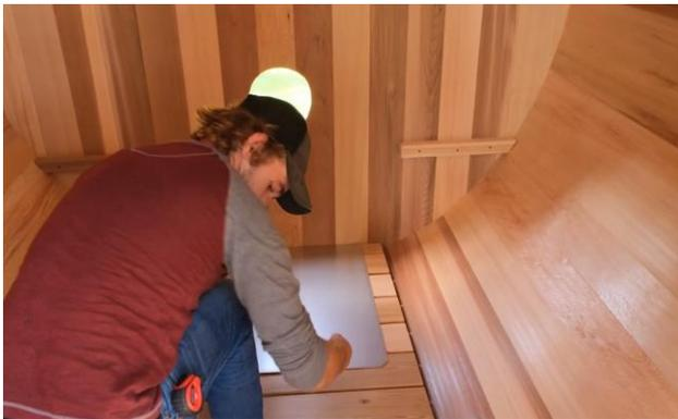
Install floor heat shield against back wall centered between the benches.
