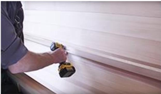
Position assembly in place and secure to sauna walls and floor using 5- 2 ½" (64mm) screws on the top and bottom rails.
