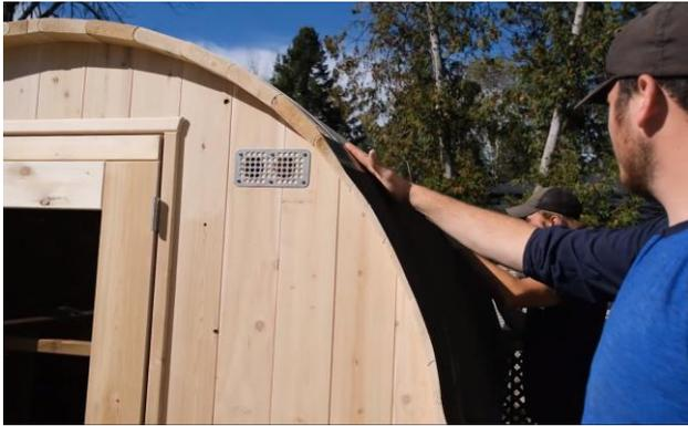
To start the installation of your bevel siding, unpeel the ice & water shield and stick it to the side of the sauna starting at the middle on one side.
