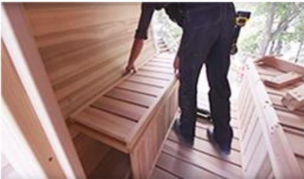
Ensure bench is flush and secure with 2 ½" (64mm) screws between the seat boards so the screws are less visible.
