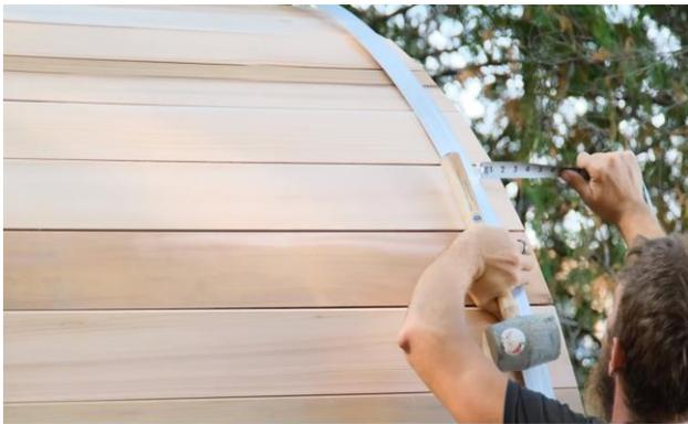
Ensure the band is 2" (51mm) from the edge of the sauna all the way around.
