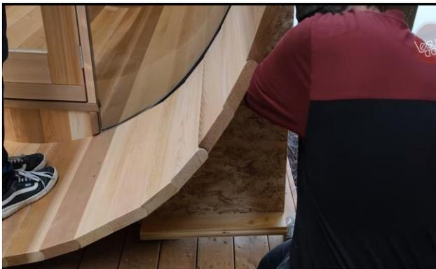
Use the wall support piece to push the wall snug into the window panel.
