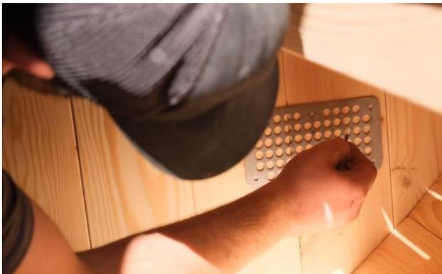
Below the bench support on the back wall, mark the vent hole position.
