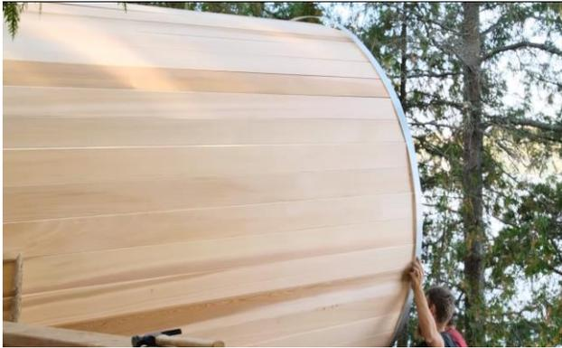
Slide the assembled band over the back end of the sauna.
