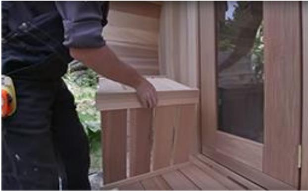
Assemble the seat and front enclosure together using 2 ½" (64mm) screws.
