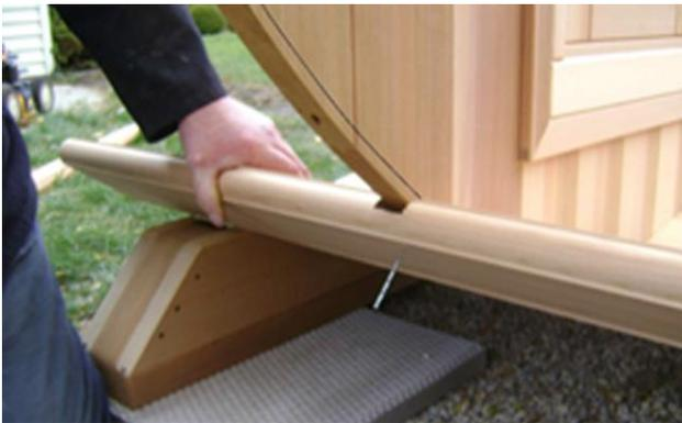
When installing the staves, tap tightly together while leaving as much of a gap as possible between stave and wall using the pencil line as a guide as in picture.
