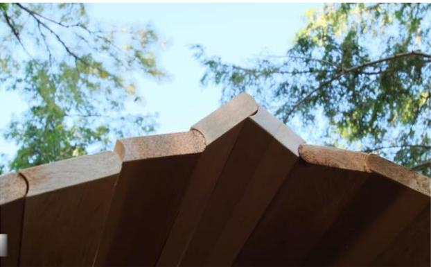
Wedge the top center stave (concave on both sides) with the last stave, to create a "V" shape.
