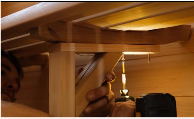
Place the bench support bracket under the seat supports and secure with 3 – 1 ½" (38mm) screws.
