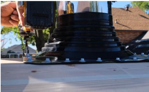
Pull the boot back down and secure with the included self sealing roofing screws 2-3" (51mm to (76mm) ) apart.
