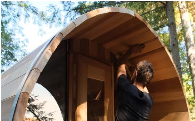
Tap out all the staves while tightening the band ensuring the staves are even.
