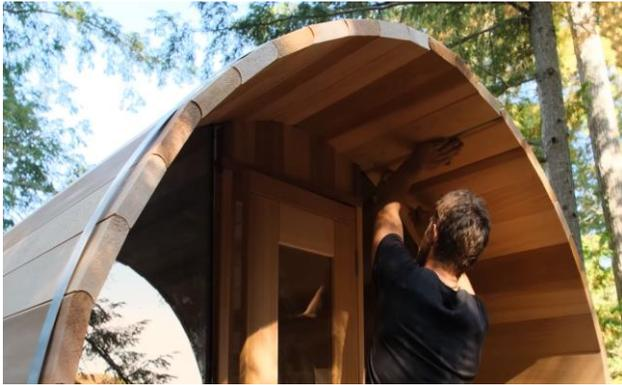
When the wall staves take on the proper shape, tighten the steel front and back bands completely.
